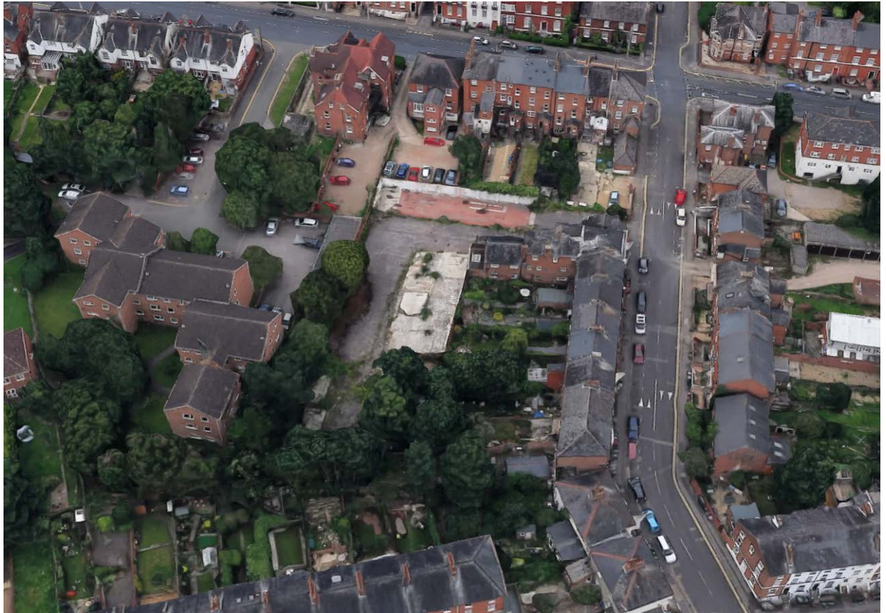
Aerial view looking west
